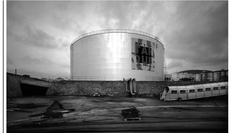
El Tanque and its site are declared a BIC (protected industrial heritage), the first in the Canary Islands
